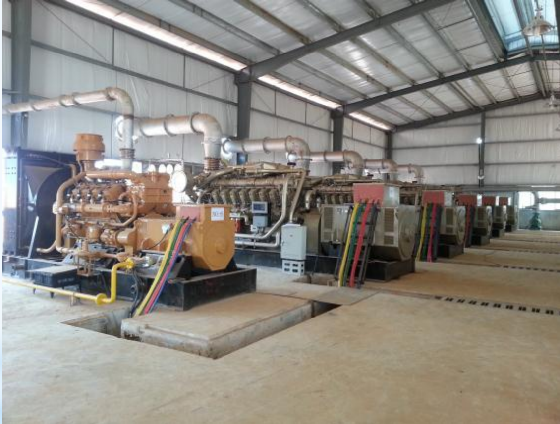
5 x 1200 kw + 1 x 300 kw genset in Nigeria
