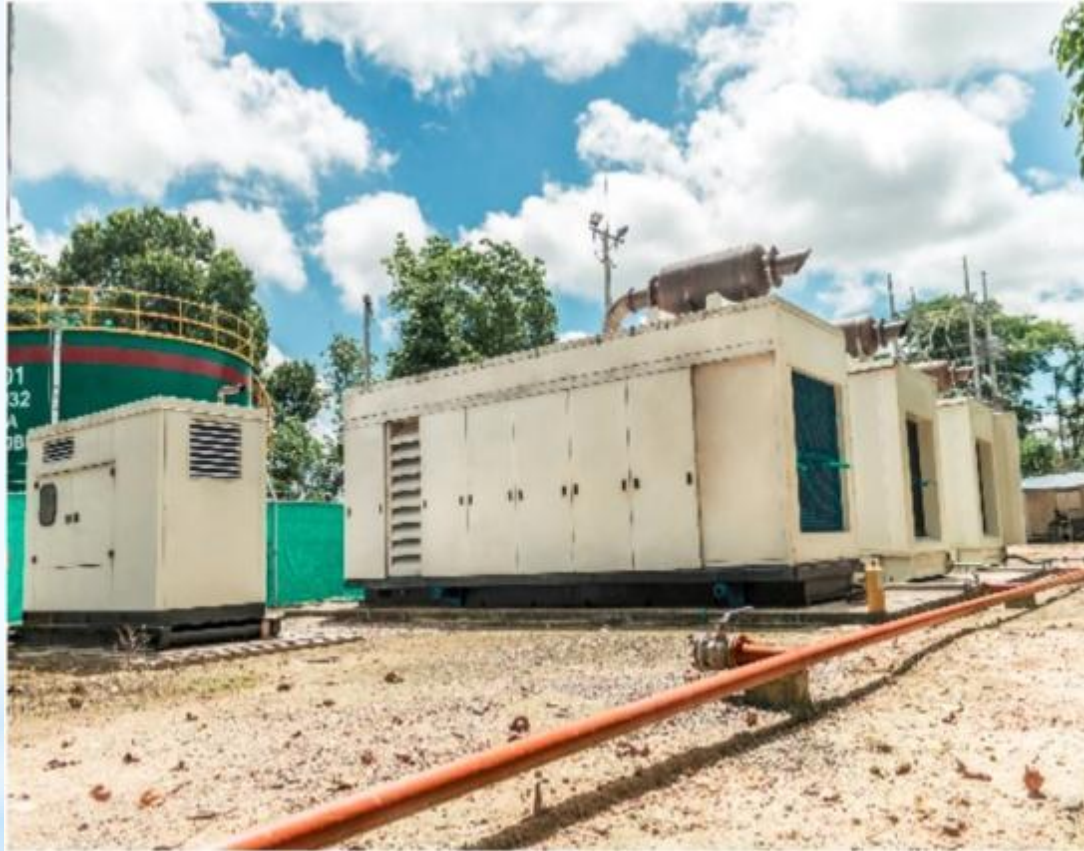
3 x 500 kw gas genset in Colombia
