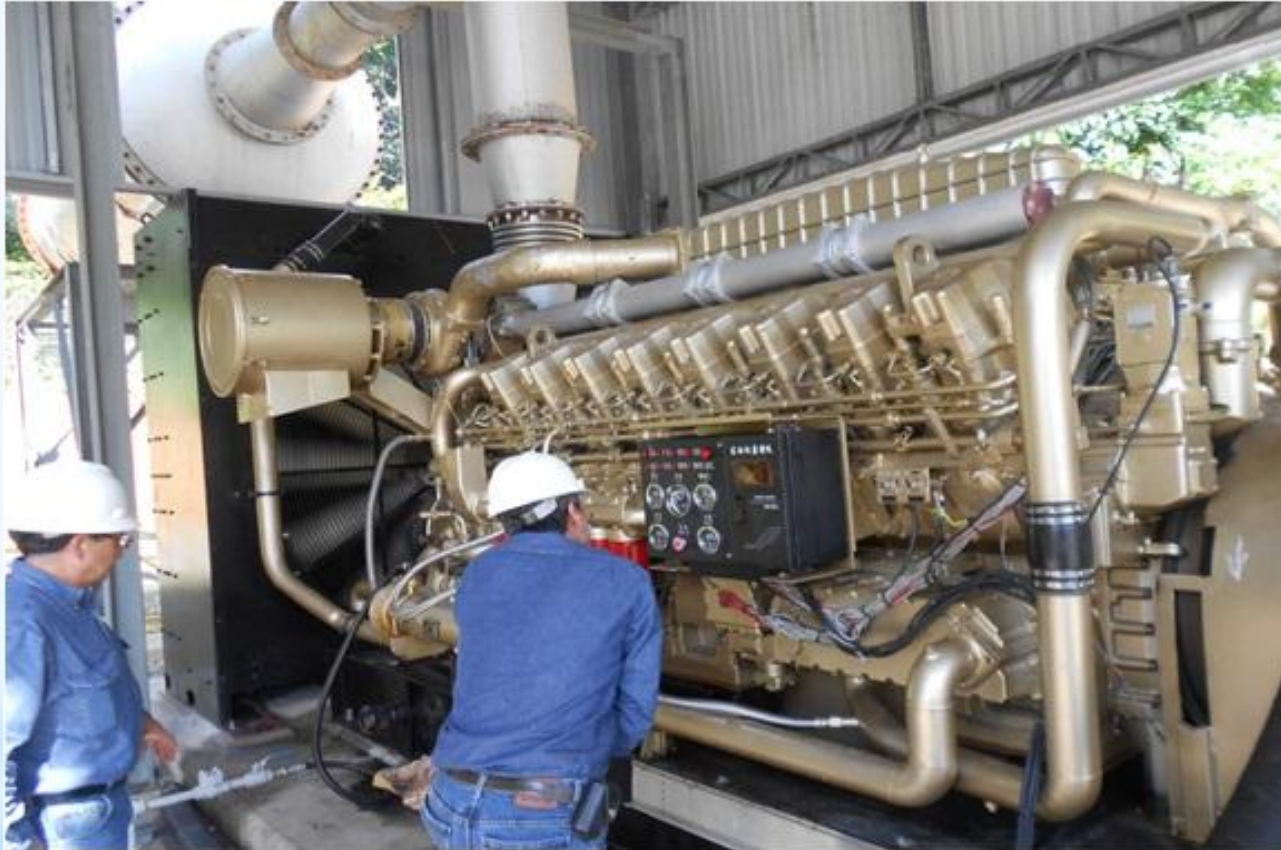
Maintenance service in Ecaudor
